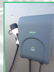
Vindu for kWh meter
